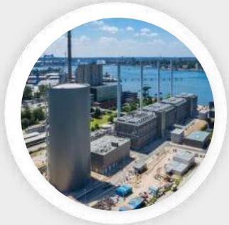
Natural Gas CHP
